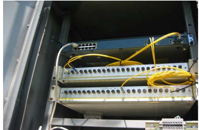
Figure 4. ODFs and switch at Nata Distribution Point
