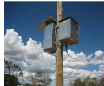
Figure 5. Outdoor enclosures at Nata distribution point (wooden on the left)
