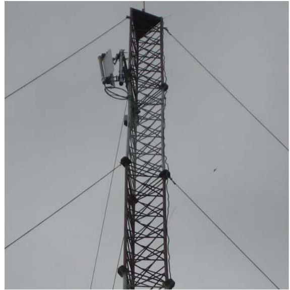
Figure 1: Access Point at Mugumu Communication Station.
