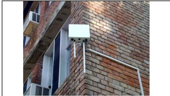
Fig 1(a) Mesh Portal connected through Ethernet
