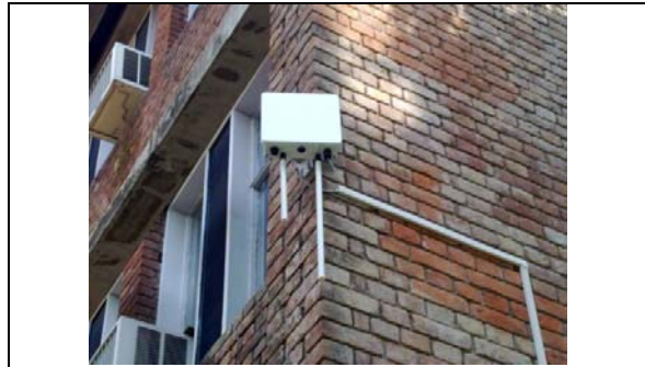
Fig 1(a) Mesh Portal connected through Ethernet
